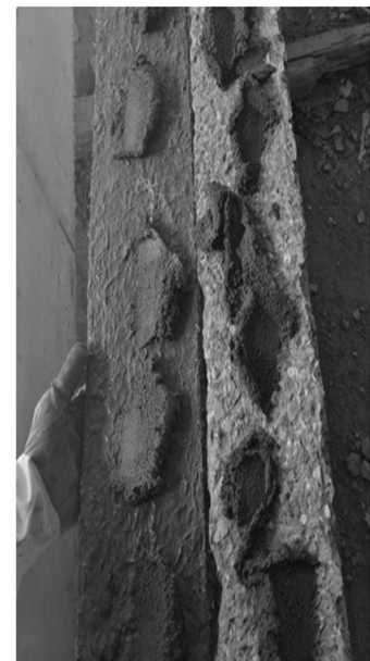
Application of the epoxy adhesive
