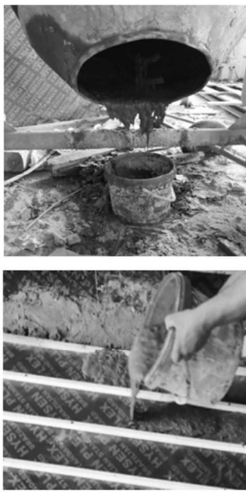
Casting of the prefabricated layer
