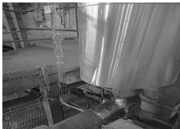
Fig. 1 Monitored section of steam pipeline in industry
